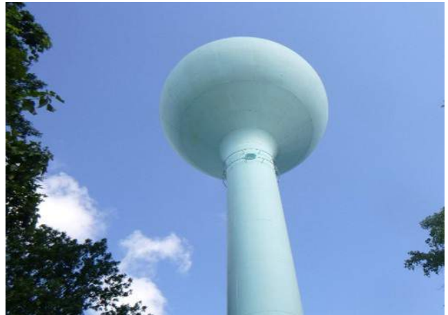
Plant No. 5 - Elevated Water Tank - Present Day
