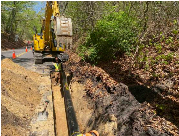
Water Main Installation along Glen Cove Road
