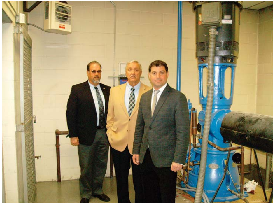
Commissioners Robert J. McEvoy, Richard P. Niznik and Michael F. Rich, III at new rehabilitated Well No. 6-2 on Berry Hill Road
