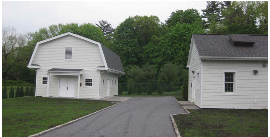
New Treatment Building (Left) and Existing Wellhouse No. 2-2 at Shutter Lane
