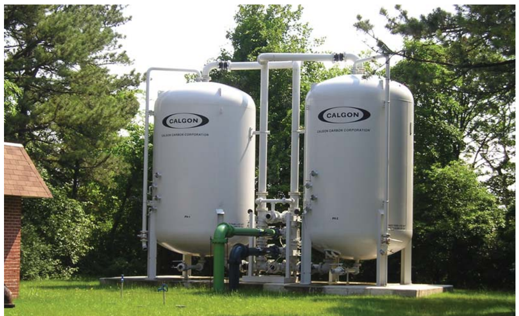
Typical Granular Activated Carbon Treatment System to be installed within Treatment Building
