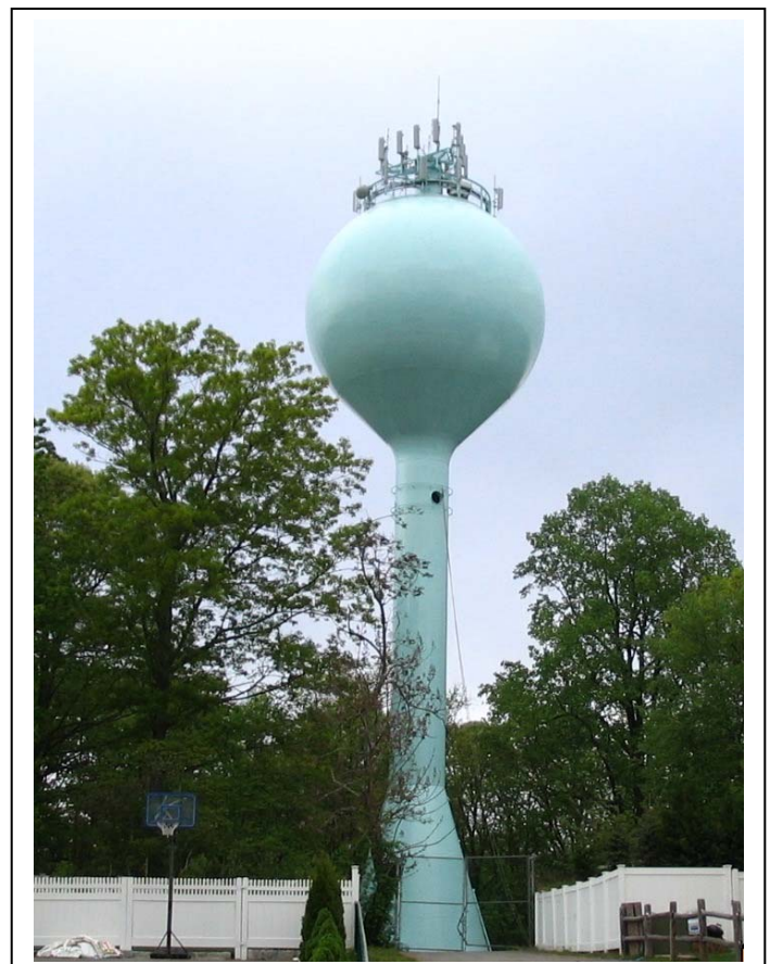
Schoolhouse Place tank after rehabilitation and repainting project.
