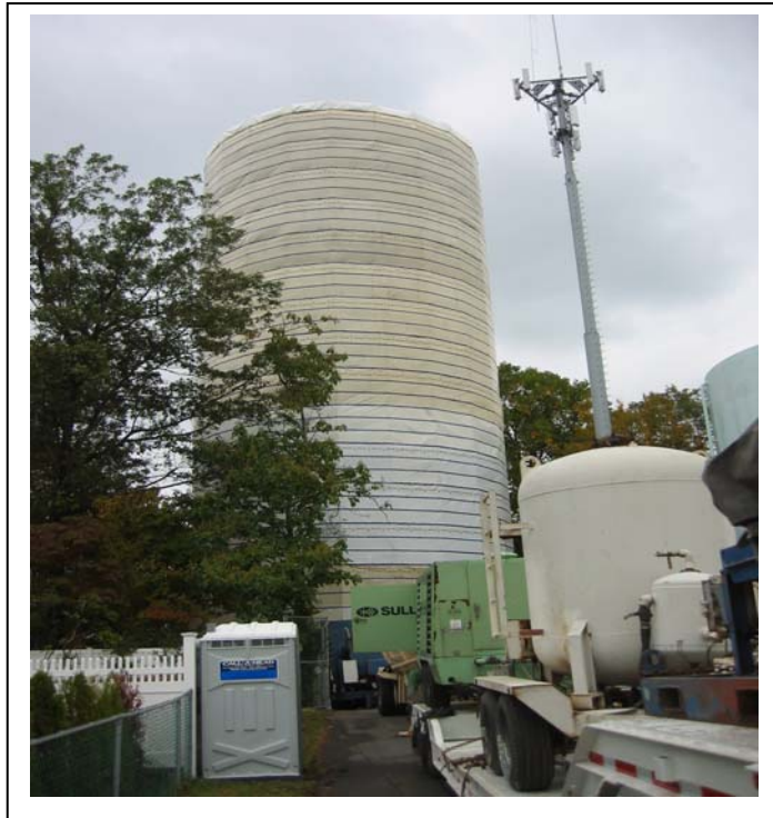
Schoolhouse Place tank under full containment during repainting.
