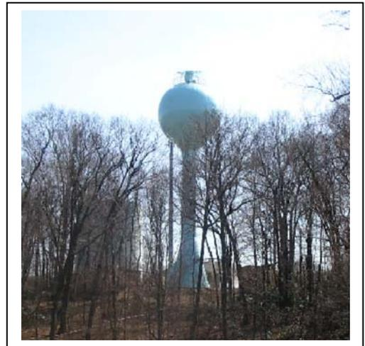
As part of this project, a contractor was hired to sandblast off the old interior and exterior painting system and replaced it with a current state-of-the-art, Health Department approved coating. In addition, we have streamlined and consolidated the cellular antennas on the tank, improving the tank's appearance. We have added safety climbing devices and equipment on the tank make it safer for our employees and contractors to work on the tank.
